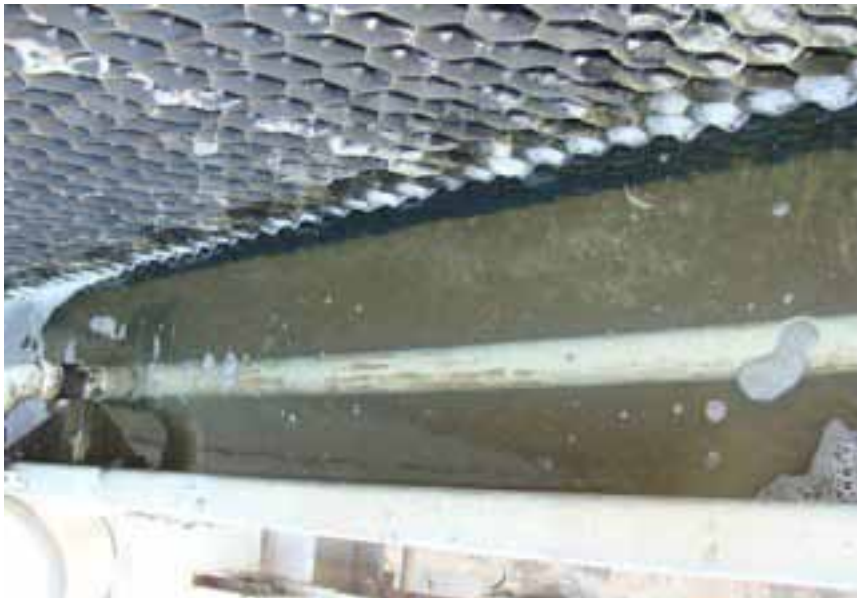
PHOTO 19. Day 16, Site E. Basin was cleaned the prior day.
