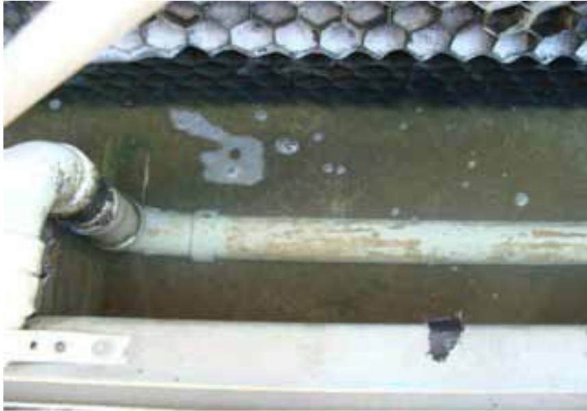
PHOTO 10. Day 16, site D. The tower was vacuumed on day 15, as part of its regularly scheduled maintenance, removing much of the dead algae and sediment.
